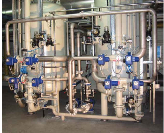
Condensate polishing line
