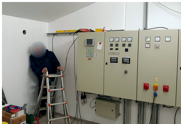
Assembly of a switchgear by our employees
