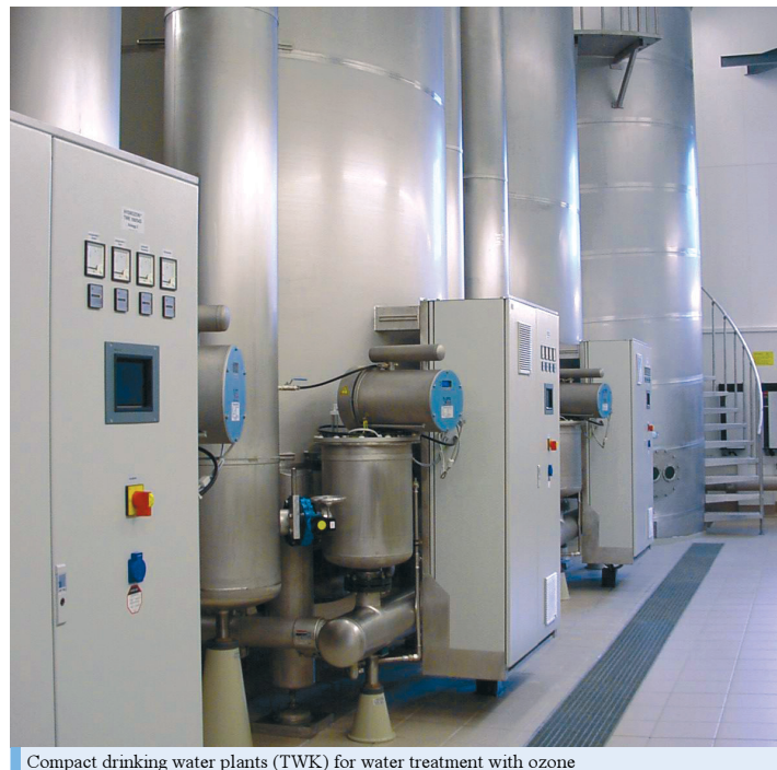
Compact drinking water plants (TWK) for water treatment with ozone
