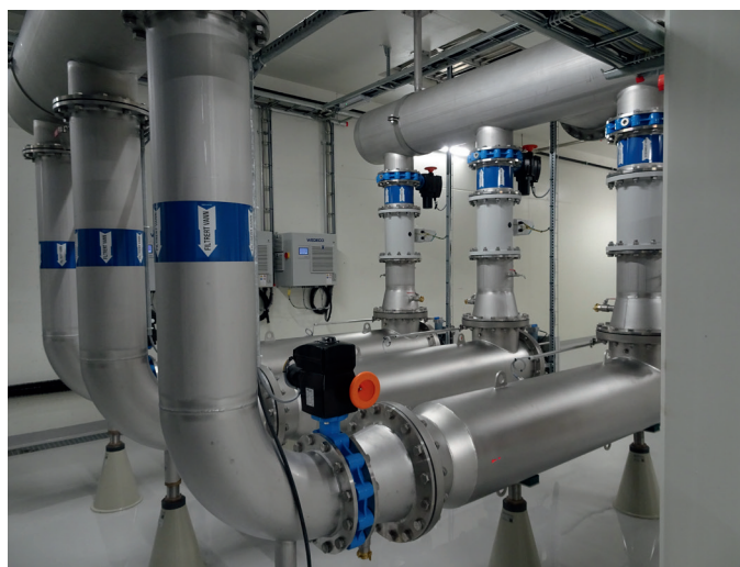
Figure 8: UV system for final disinfection
