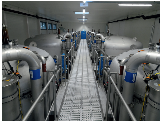
Figure 6: Top operating level of the ten filter systems
