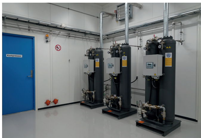
Figure 3: PSA systems for oxygen generation
